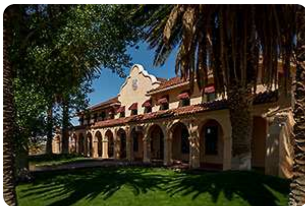
Kelso Depot and Visitor Center
